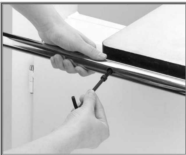
Figure 22. Securing rail with cap screw.
